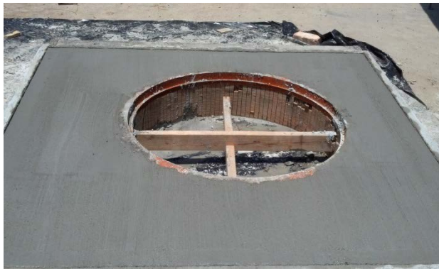
Above: Junction Box Cast-in-Place Concrete Lid
