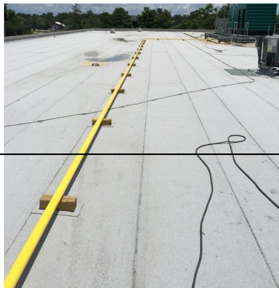
New Modified Bitumen Roof System
