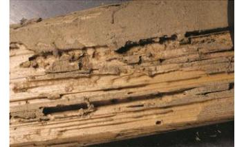
Formosan termites are an especially robust, destructive species with large colonies. Walls of infested buildings may contain carton nests that hold enough moisture to allow the colony to live entirely above ground, sometimes causing bulging walls.
