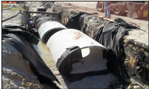
**Installed 45"x73" RCPA drainage culvert**
