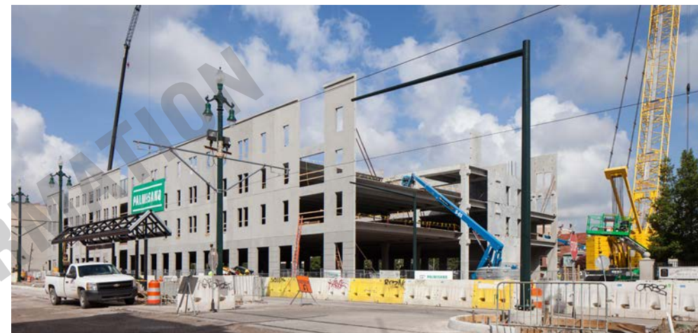
Homewood Suites precast panels installation
