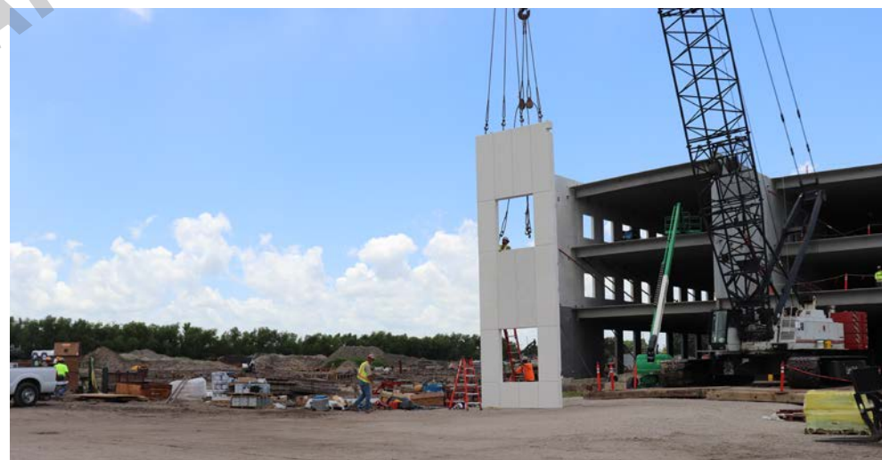
Kenner Discovery Health Sciences Academy precast panels in progress
