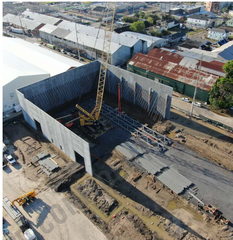
Precast panels being installed on Second Line Stages new production studio
