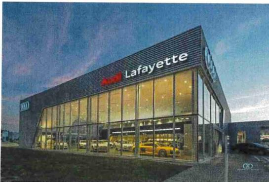
**Audi Dealership, Lafayette, Louisiana** - 40,000 square foot multi-story steel and concrete building consisting of mezzanines, offices, meeting rooms, and show rooms. Structure is supported by a soil supported foundation, steel framing designed for gravity and lateral loads, elevated concrete decking designed to span between structural steel joists and provide rigidity throughout building. Construction cost \$7,000,000.00.
