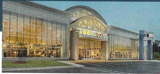
**Rooms To Go, Covington, Louisiana** - Analysis and design of moment and shear bracing, column, and girder connections for new 37,000 square foot steel framed retail building. Calculations included both bolted and welded connections using W, tube, and pipe sections, as well as, truss members.
