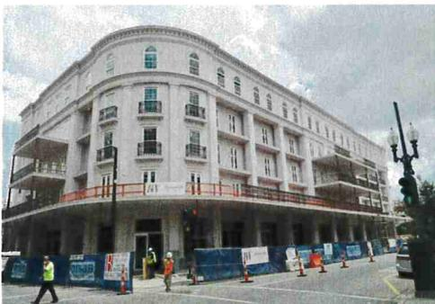
**700 and 640 Magazine Street Handrails, New Orleans, Louisiana** - Multi-story historic building requiring new balcony handrails meeting current building code. Analyzed and designed connections for multiple types of steel railing and handrail configurations.
