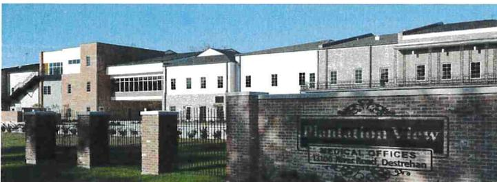
**Plantation View Medical Offices, Destrehan, Louisiana** - 65,000 square foot, three story steel and concrete building, supported by deep foundation, structural and light gauge steel framing, elevated concrete. Construction cost \$6,000,000.00.
