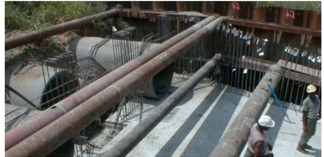
The main scope of this project consists of new cast-in-place concrete boxes of varying sizes supported on a jet grouted foundation. Four culvert types were designed: an 8-foot by 6-foot culvert 2,350-feet in length (split into 50-foot monoliths), a 10-foot by 8-foot culvert 2,550-feet in length (split into 50-foot monoliths), a 12-foot by 10-foot culvert 2,348-feet in length (split into 50-foot monoliths). Additional culverts were also designed as transitions between the four culvert types.
