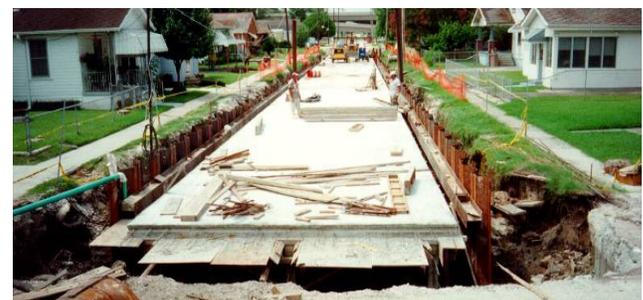
The work on Avenue B consisted of replacing existing major subsurface drainage system with new concrete pipe varying in size from 15 to 54 inches in diameter. The limited space along the corridor required major utility relocations, complete roadway removal and replacement and detailed excavation plans to protect adjacent residences within 20-feet on either side of the
