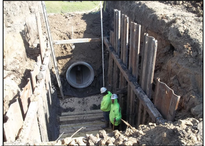
Installation of 42" RCP Culvert on Myrtle St. Outfall between Mistletoe St. & Canal No. 6
