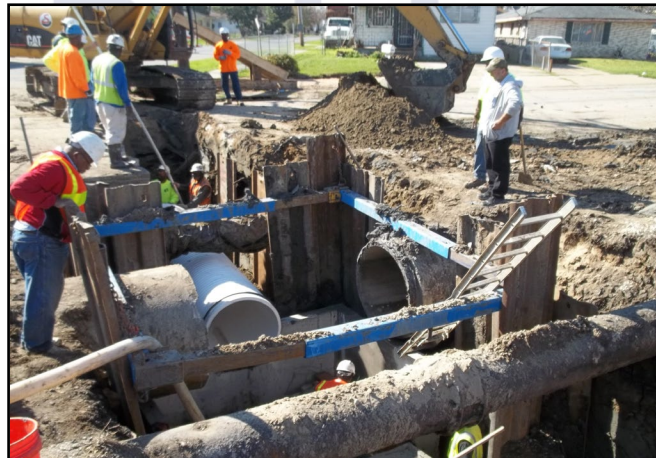
Installation of 36" PVC Pipe across Mistletoe Street on Meadow Street Outfall
