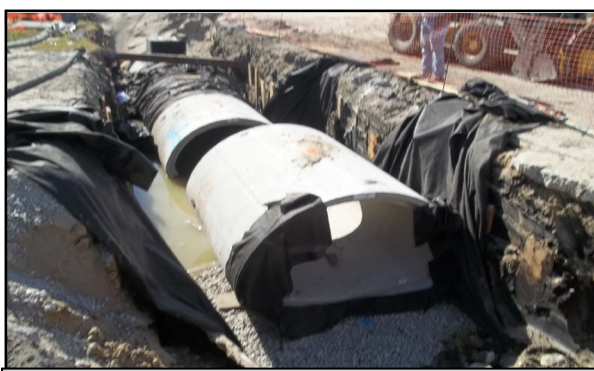
Installed 45"x73" RCPA drainage culvert
