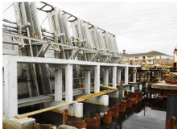
CITY BARN PUMP STATION BAR SCREENS - HMGP FUNDED
