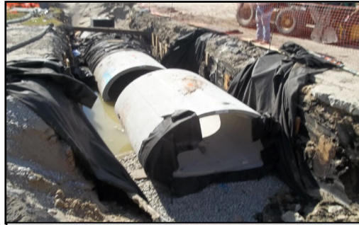
Installed 45"x73" RCPA drainage culvert
