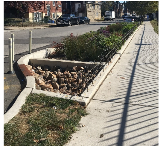
Green City, Clean Waters, Philadelphia, PA. A roadway shoulder is transformed into a stormwater management facility providing water quality and water quantity treatment for the surrounding roadway and sidewalk areas.
