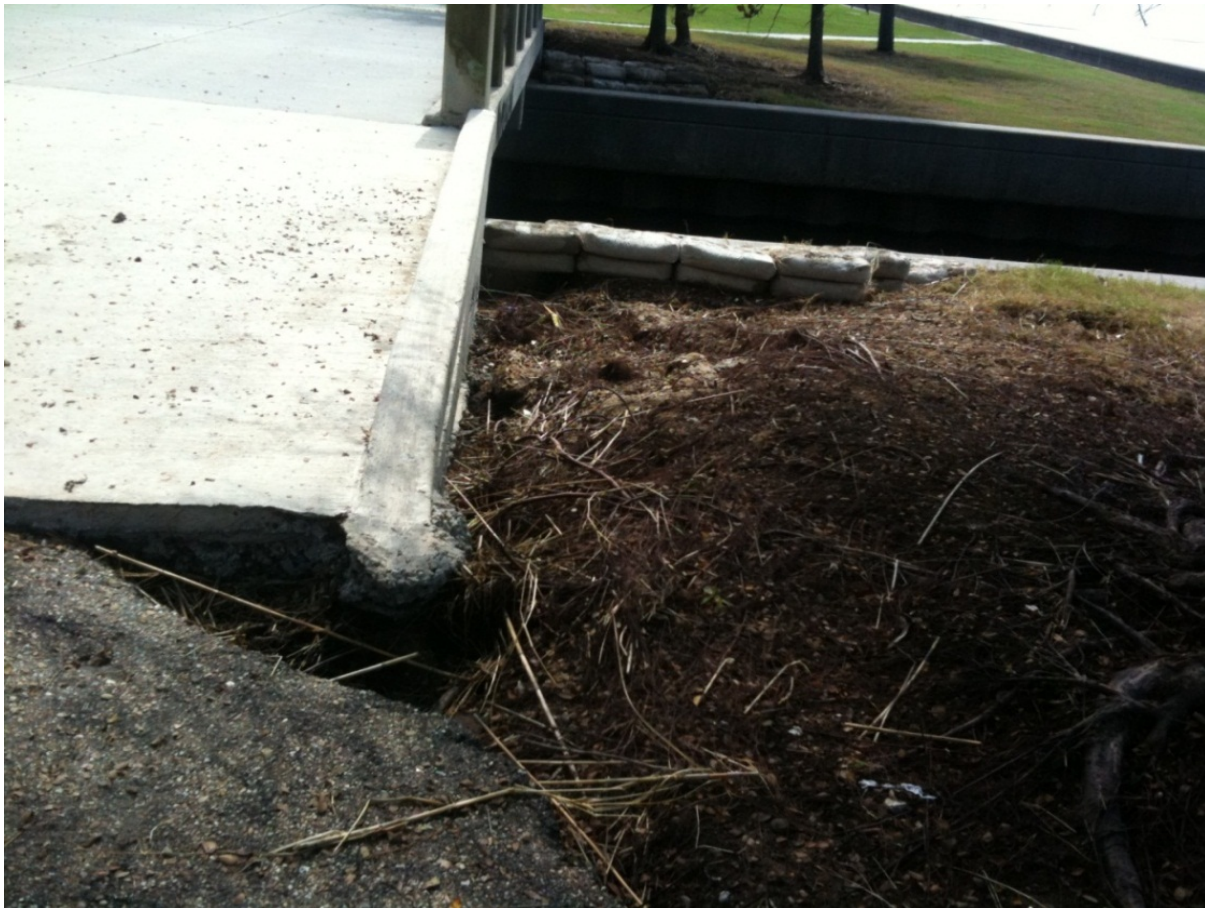
Figure 1. Asphalt Pavement –Base failure
