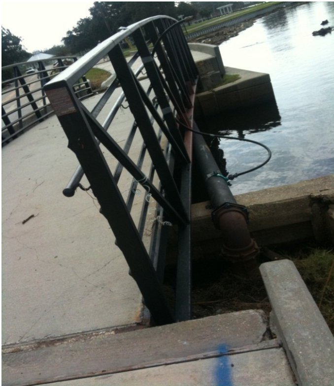
Figure 3. Bridge Detachment
