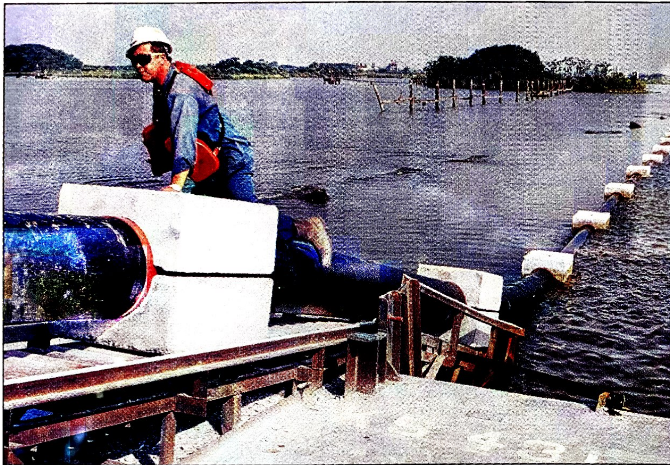
The pipe is floated onto the Barataria Bay Waterway during the joint fusion process occurring on the barge.
