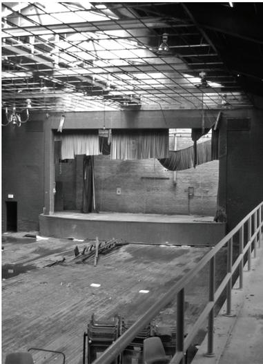
The historic Buras Auditorium suffered significant damages as a result of Hurricanes Katrina and Rita. This included collapsed roof sections, completely destroyed wood floors and joists, ruined building systems, destroyed interior finishes among many other items.
