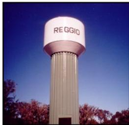
**Elevated Water Tank in Reggio, LA:** Design, bidding, construction administration, and resident inspection for a 500,000 gallon, elevated hydropillar water tank with fluted steel columns.
