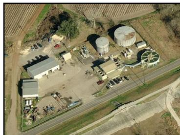
**Convert Water Treatment Plant:** Design, bidding and construction administration to upgrade the existing 1 MGD plant to 1.7 MGD, and repairs to the water intake pipe. The design provided solids contact clarification and rapid sand filtration. A hydraulic analysis was conducted in order to determine the capacity and head requirements of the high service pumps.
