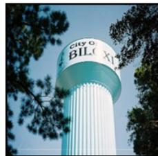
**Elevated Water Storage Tank No. 2, Cedar Lake Road & I-10:** Design, bidding, and construction administration for a **one (1) million gallon elevated water storage tank.**
