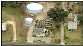
**Edgard Water Treatment Plant:** Design, bidding and construction administration to upgrade the existing 0.45 MGD plant to 1 MGD. The design provided raw water pumping, solids, contact clarification, rapid sand filtration, backwash, pumping, clearwell storage, chemical feed, chlorination, transfer pumping, high service pumping, raw water and high service flow measurement, wastewater treatment and pumping, standby power generation, and site improvements.
