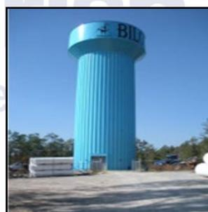
**Elevated Water Storage Tank No. 4; Woolmarket:** Design, bidding, and construction administration for a **one (1) million gallon elevated water storage tank.** N-Y utilized the EPA.Net Program to model the water system for the Woolmarket area to confirm the capacity and elevation of the water tank.
