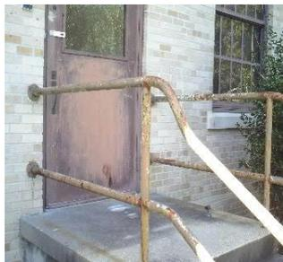
Results included LBP identified on the exterior wood doors, door frames, and walkway hand rails; and lead-based coatings identified on the ceramic wall tile located in the restrooms and on yellow storage cabinet in one room. Terracon provided recommendations for removal of the LBP in accordance with regulatory guidelines.
