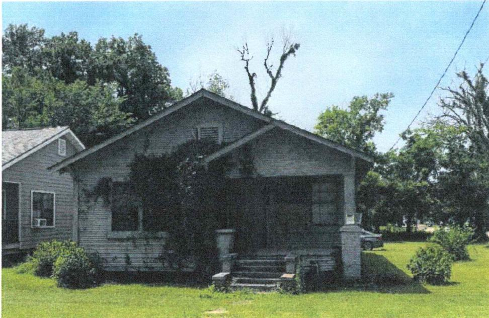
An inspection for asbestos-containing materials was conducted for this structure by Petroleum and Automation Consultations, Inc. (PAAC). The Asbestos Bulk Sampling Report issued by PAAC, under the "Summary of Findings," reported that there was no detectable asbestos (greater than 1%) for this structure. Bidder is referred to the Asbestos Bulk Sampling Report included herein as Exhibit "C" for further information of the asbestos testing and test results.
