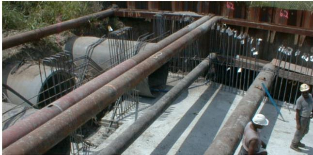
The main scope of this project consists of new cast-in-place concrete boxes of varying sizes supported on a jet grouted foundation. Four culvert types were designed: an 8-foot by 6-foot culvert 2,350-feet in length (split into 50-foot monoliths), a 10-foot by 8-foot culvert 2,550-feet in length (split into 50-foot monoliths), a 12-foot by 10-foot culvert 2,348-feet in length (split into 50-foot monoliths). Additional culverts were also designed as transitions between the four culvert types.
