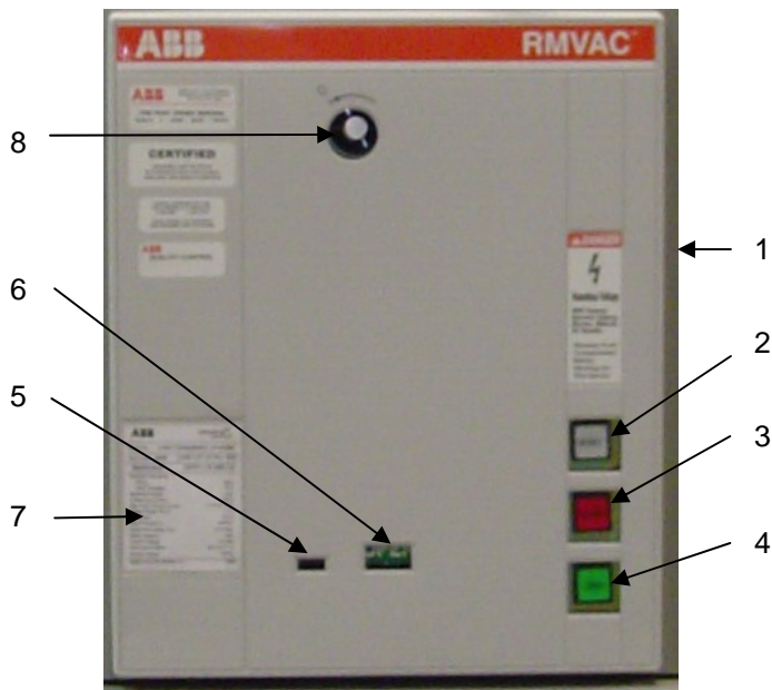
Figure 2a: Circuit breaker front with controls
