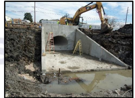
Wedmore Drainage - West Culvert
