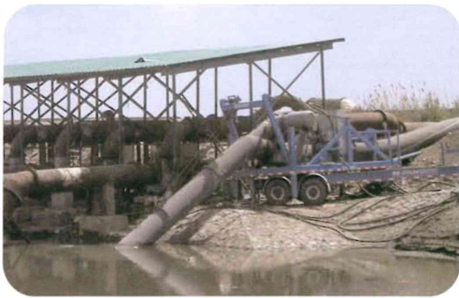
30" Mobile pump bypassing permanent pumps.
