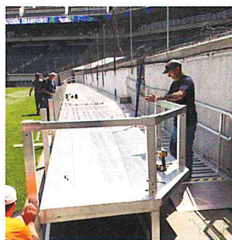
Individual platform components were manufactured in AAE's shop and delivered for on-site install
